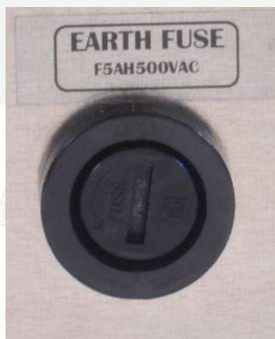
Figure 11: earth fuse housing
